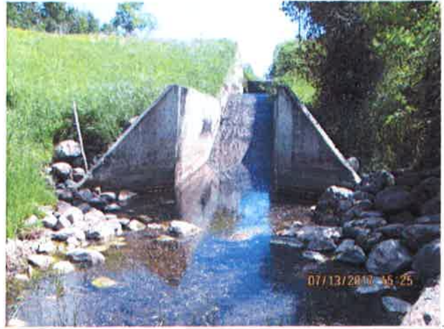
North Branch Drop Structure – JD 31
