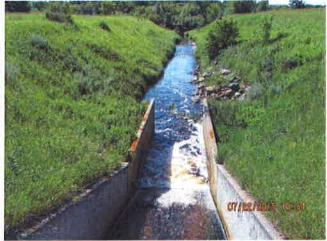
North Branch Drop Structure
