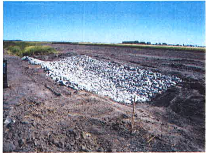
Grade Stabilization – Springbrook #10
