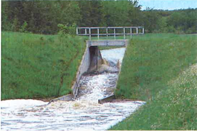
North Branch drop structure – SD 84
