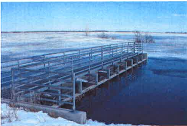
Outlet Structure at Ross #7 Impoundment
